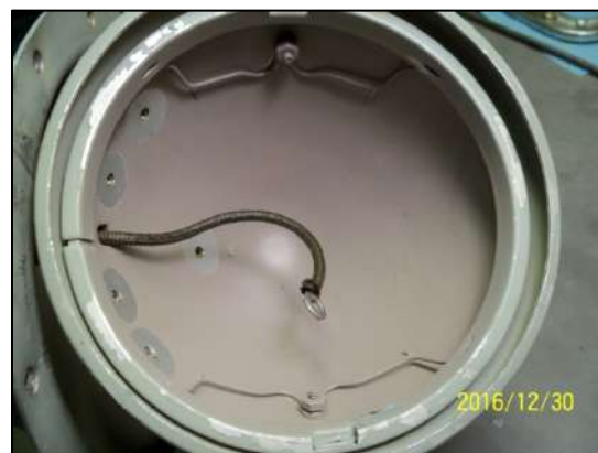
Lamp housing back shell ready to extract with mounting screws and washers removed.
